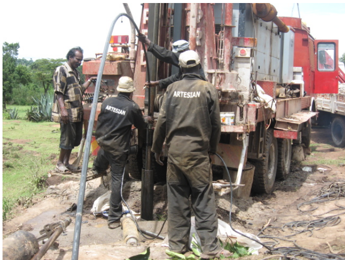
Drilling in progress at Changina shallow well site.
